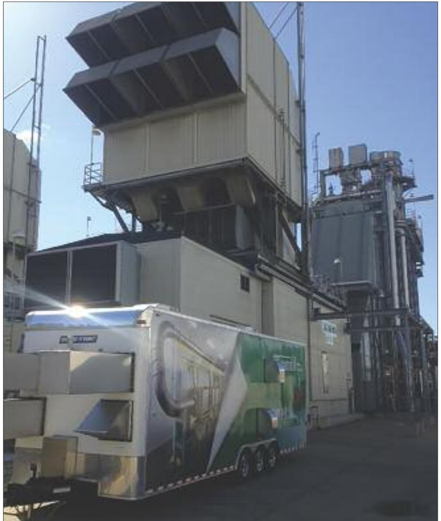
*A mobile laboratory located by the operator GT inlet. It allows up to four different filter combinations to be run side-by-side and monitored.*
